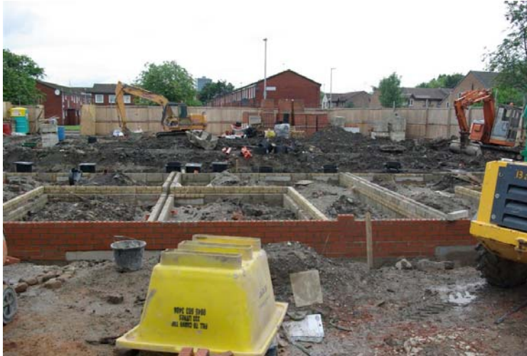
Building Site where Tilted Falcon used to be, Kincardine Road
